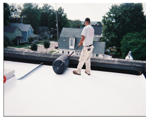
Apply pressure to the top surface of the membrane to ensure contact with a roller (not to exceed 150 lb/68 kg)
