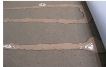
Close up of 12" Bead Spacing
