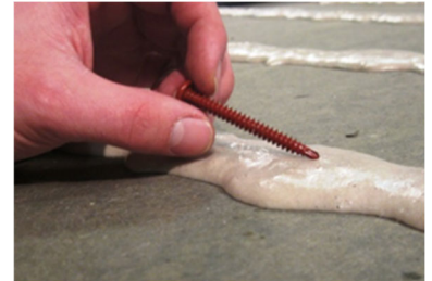
STEP 3: Tack-free stage – ready for application of UltraPly TPO XR Membrane (after 5 -7 minutes)
