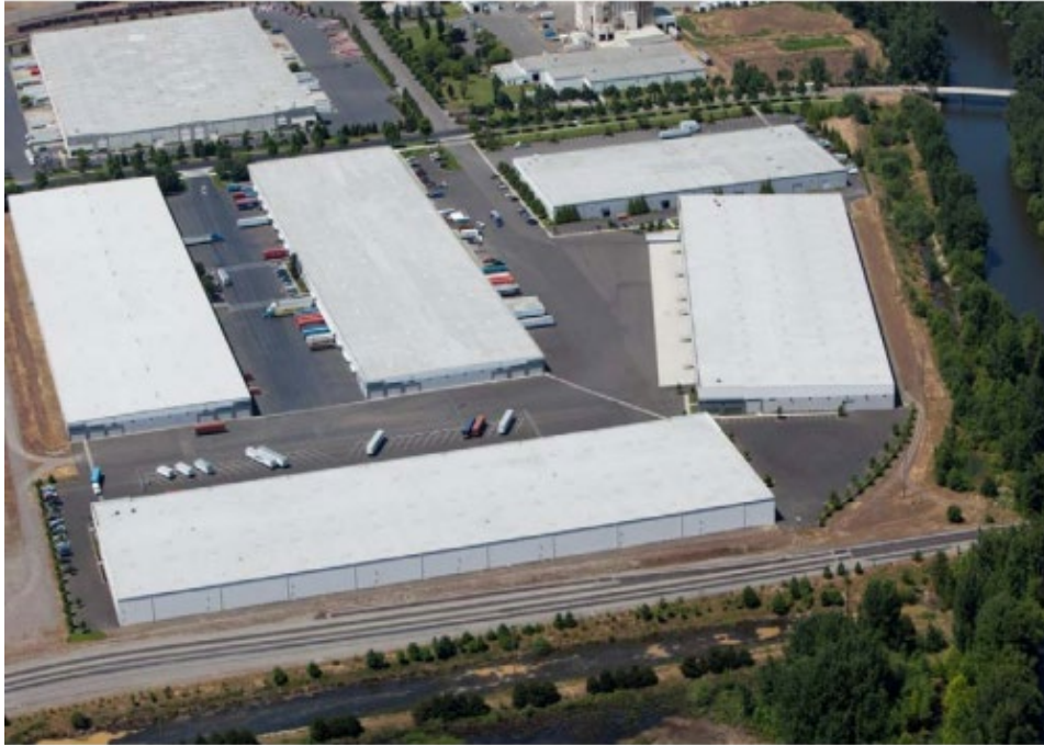
Low-slope roofing membrane of a built-up roof hot-mopped (BUR).
