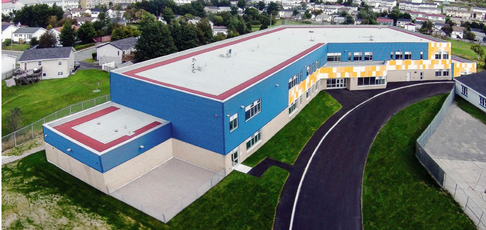
Low-slope roofing membrane of a built-up roof (BUR).
