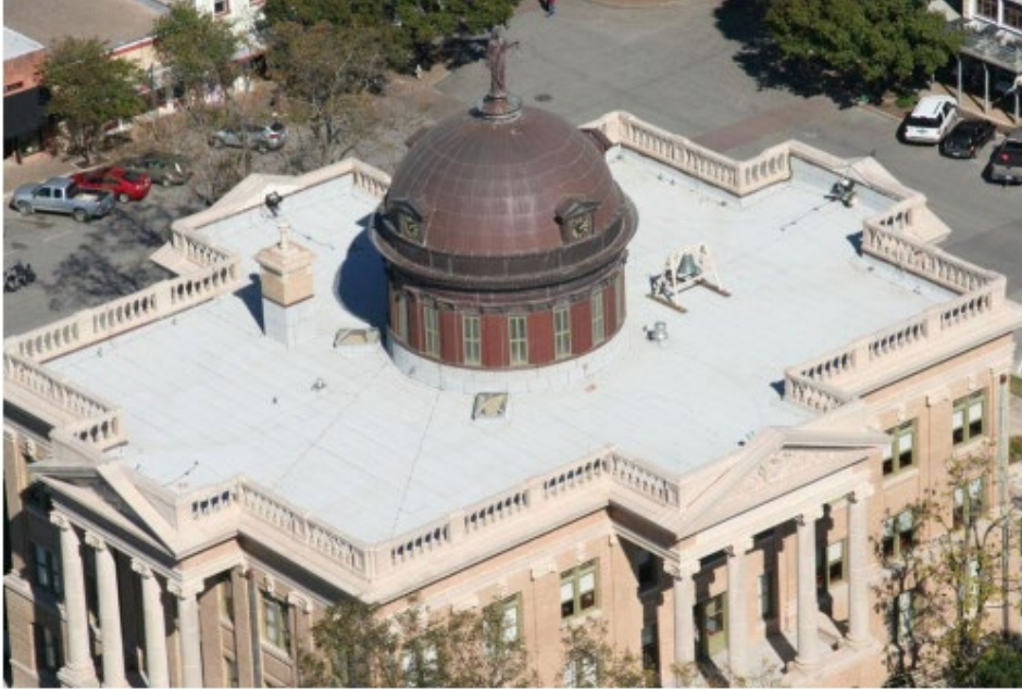
Low-slope roofing membrane installed using a propane torch and consisting of an APP-modified bitumen cap sheet and base sheet.
